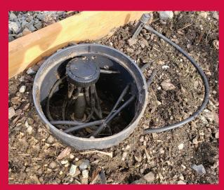
SHRUBBLERS: manifold that supplies water from the main pvc irrigation lines to the shrubblers, and a typical shrubbler in operation. Photos Ken Sheppard.
