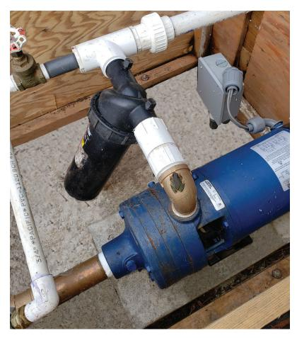
ABOVE: photo of the pump and filter, complete with a resident pumphouse frog. BELOW: a commercial self-cleaning strainer. Photos Ken Sheppard.
